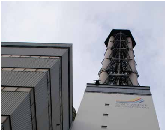
Image 5 Emblem: The tower has been seen as Duisburg's emblem since 1967. The three flues and the elevator tube in the middle represent an impressive eye-catcher when lit up by green floodlights at night.
